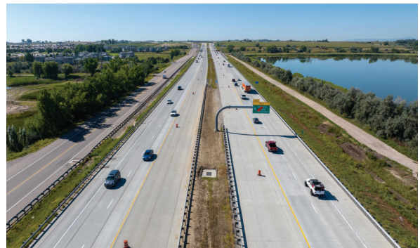
Photo courtesy of Colorado Department of Transportation
